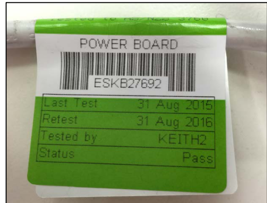
Example of an electrical testing tag
