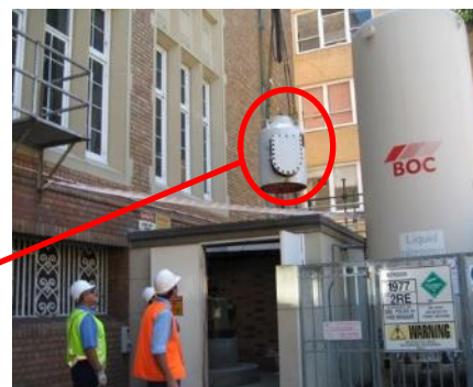
Lifting the containment vessel.
