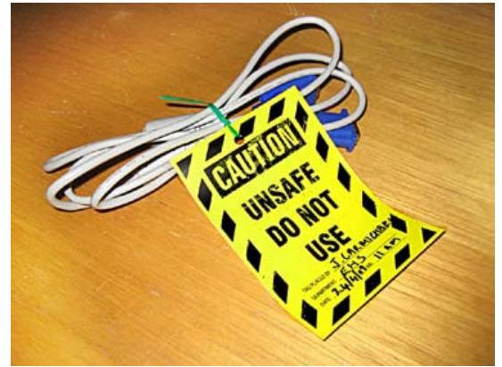
Damaged electrical cable tagged out
